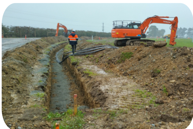
Trenches for cabling at Lauriston Solar Farm during construction
