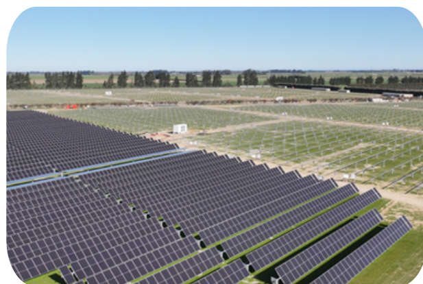
Solar farm with some panels installed and some yet to be installed
